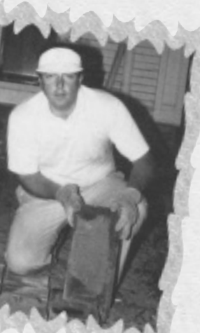
Members, including Jeff Chalmers, worked hard one Saturday in 1988 to install a brick patio in the gardens of the House.
